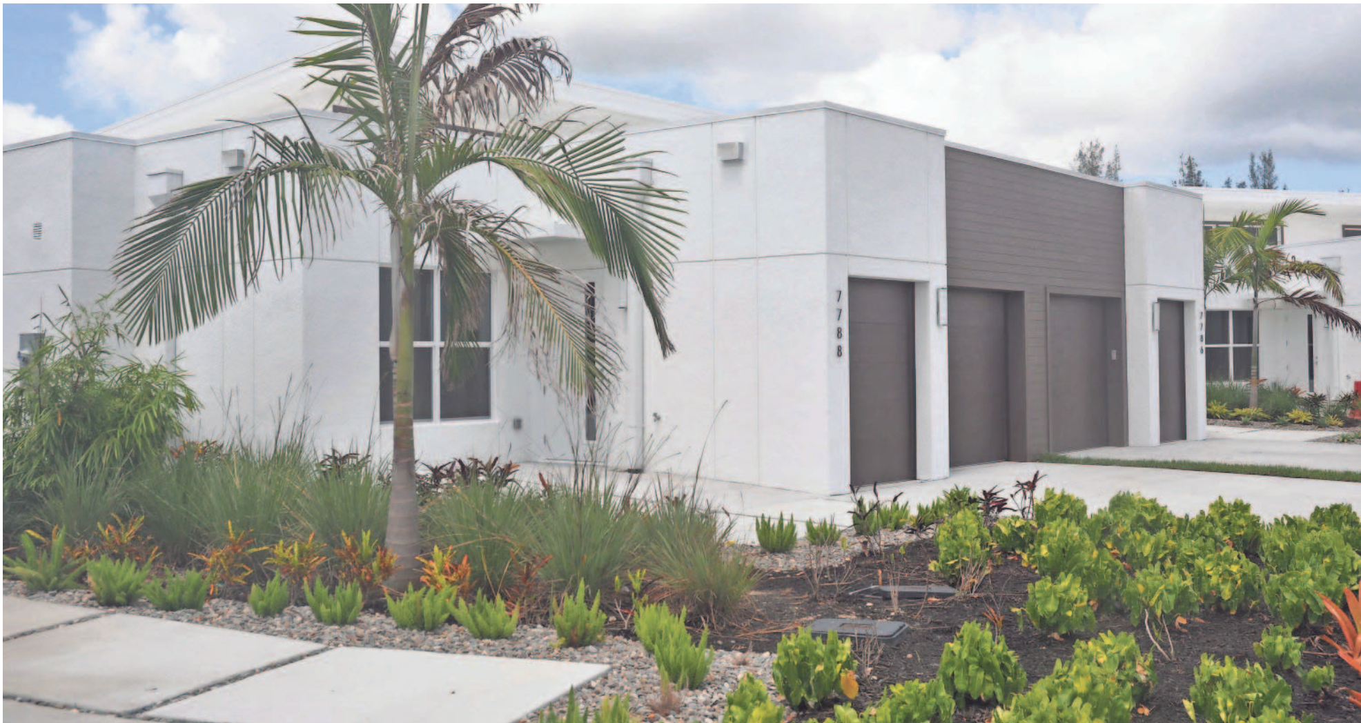
There are 28 cottages (shown) and 272 apartments in the independent living section of Amavida. PHOTOS BY ANDREA STETSON
