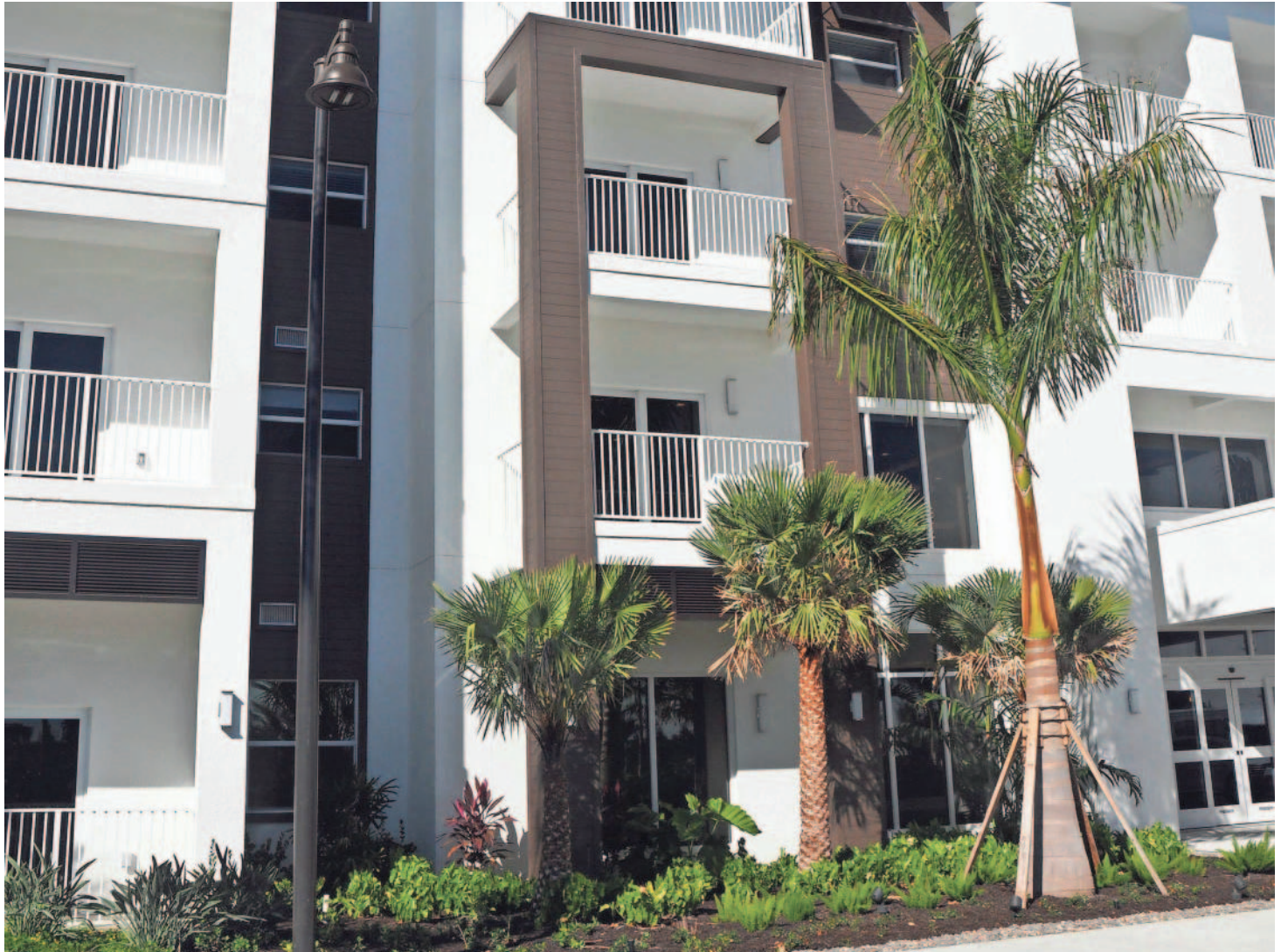
The independent living section of Amavida, which consists of apartments (shown) and cottages, just opened for residents to move in last week. PHOTOS BY ANDREA STETSON
